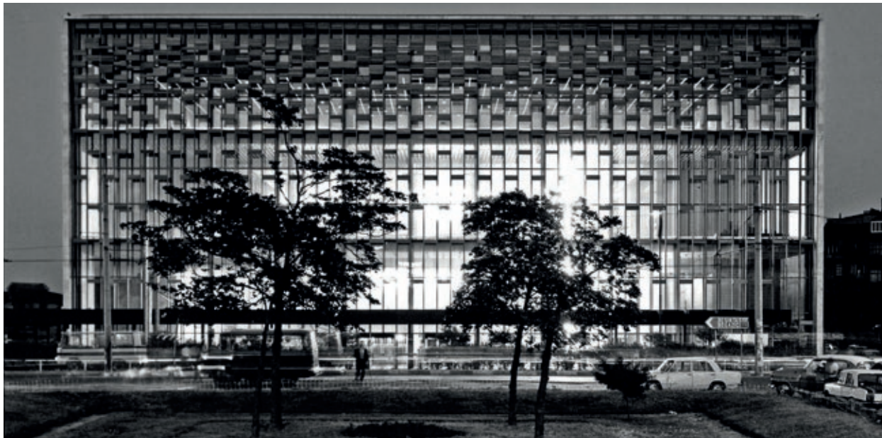
Originally built in 1946 as the "Opera House," and later transformed in the 1960s as the Cultural Center, AKM was designed by Dr. Hayati Tabanlıoğlu
